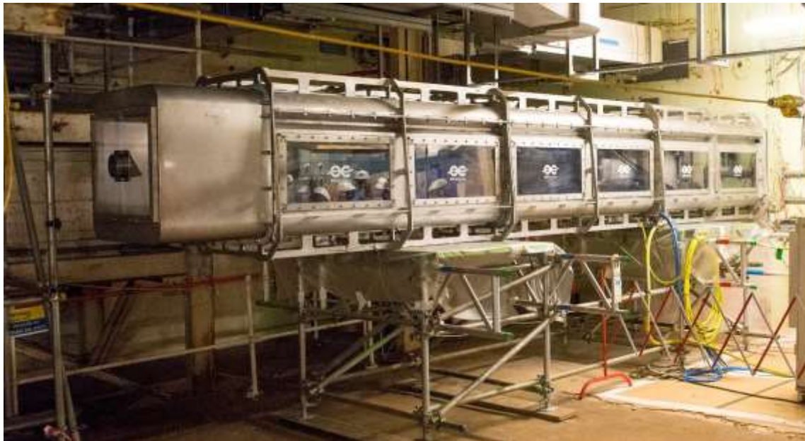
Figure 3: LaserSnake containment housing, on site at Sellafield
